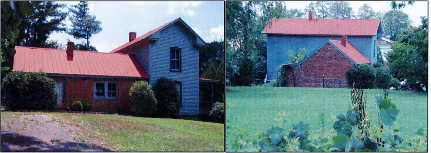
Figure 6. Rierson House—north side elevation at left; east rear elevation from rear of backyard and lot at right
