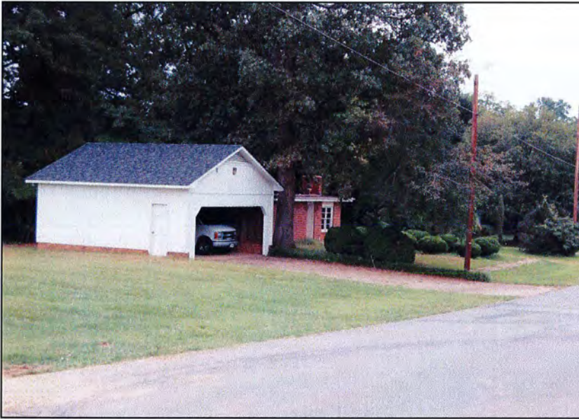
Figure 17. Looking northwest from junction of Summit Street and 6th Street toward garage and front elevation of 511 Summit Street at northern edge of Summit Street Historic District
