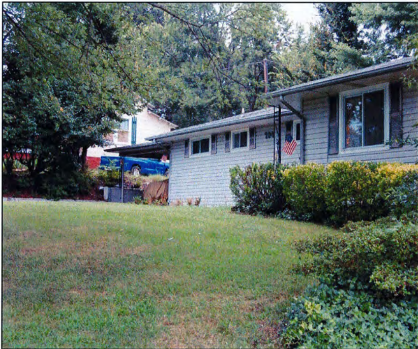
Figure 27 Looking northeast from junction of Main and 7th at late twentieth-century house at right and J. Will Wall House at left
