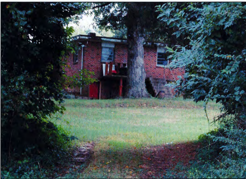
Figure 16. Looking east from High Street (alley) running along rear of Rierson House lot toward back elevation of 511 Summit Street (north of Summit Street Historic District)
