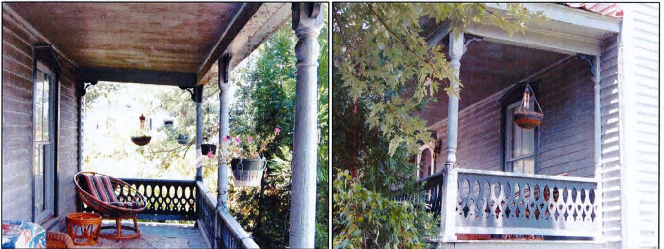
Figure 5. Rierson House: porch details
